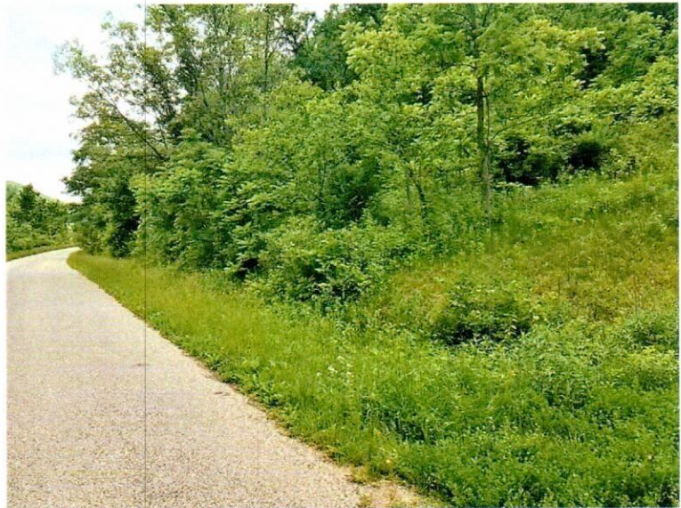
A view of the road frontage.
